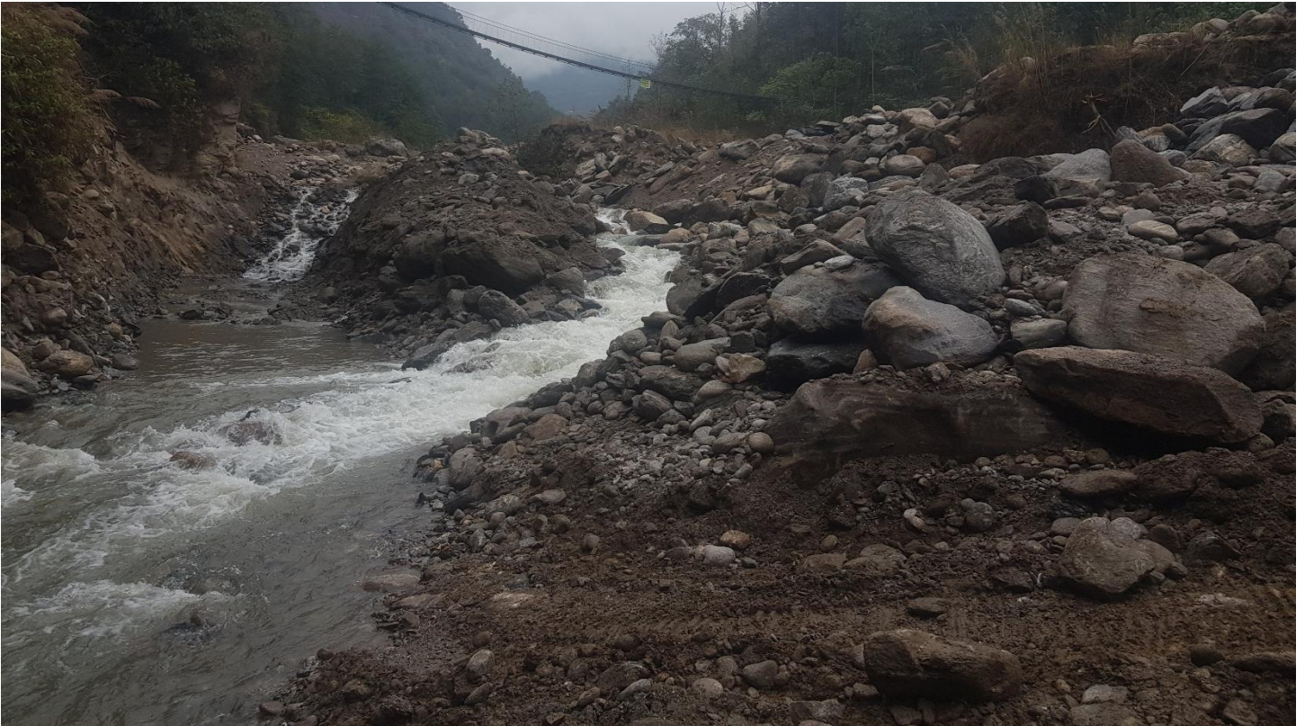
Figure 11: first stage river diversion
