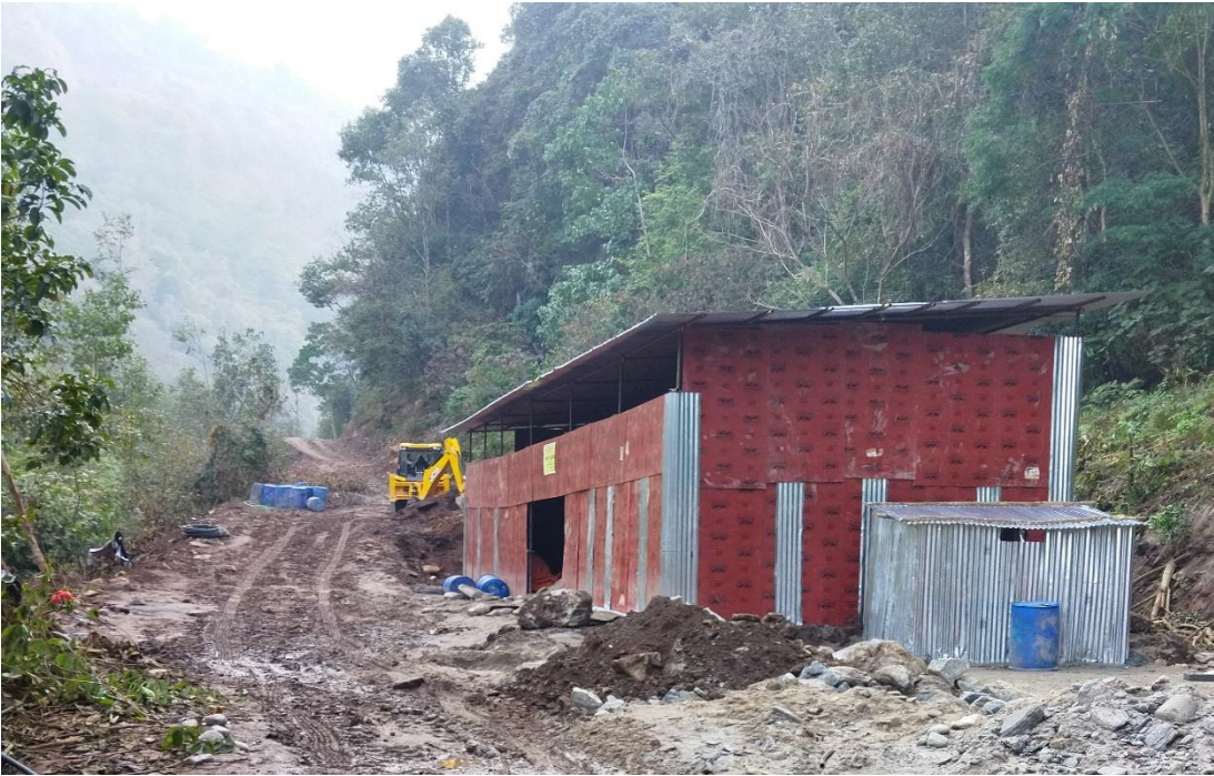
Figure 3: Labour camp at headworks
