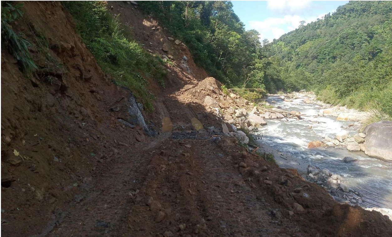
Figure 1: Access road to Headworks
