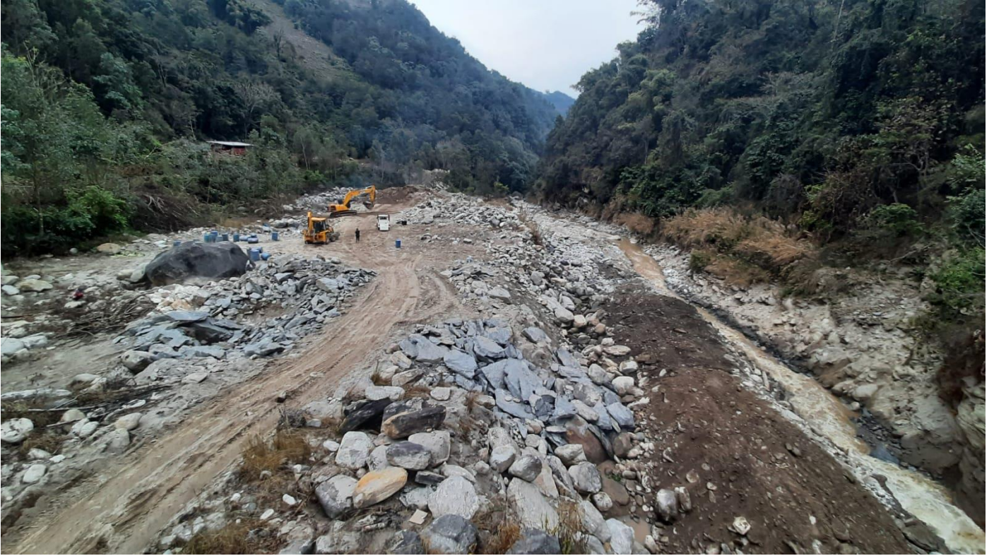
Figure 11: first stage river diversion
