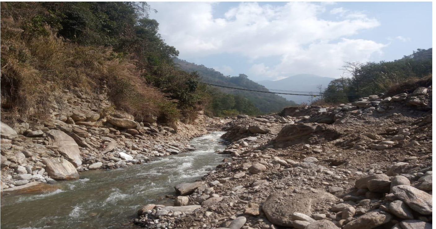
Figure 13: Cofferdam and Diverted river to right side
