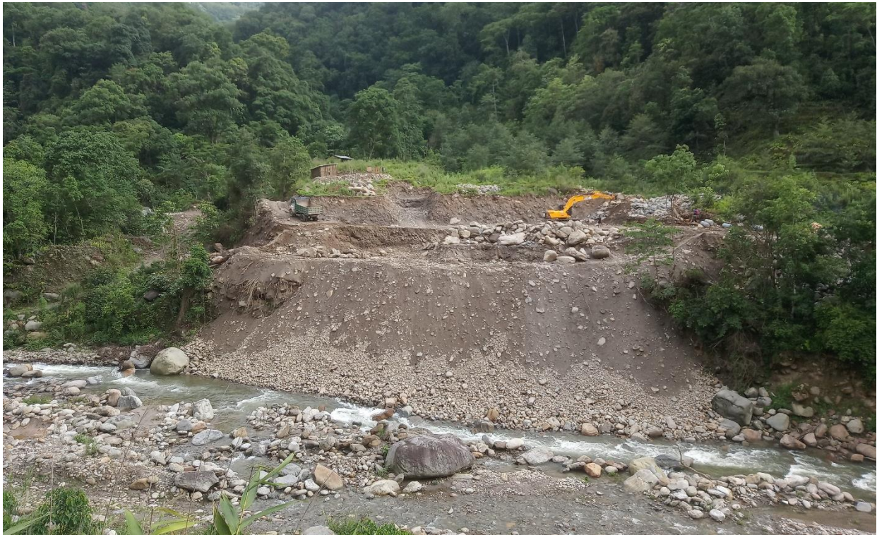
Figure 15: Excavation for Powerhouse Structures
