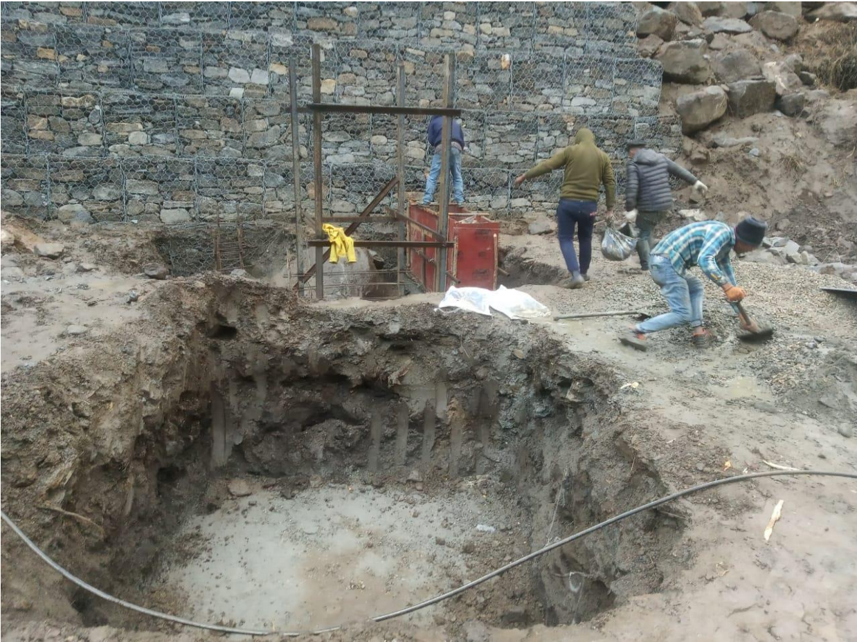
Figure 14: Crusher Plant foundation works
