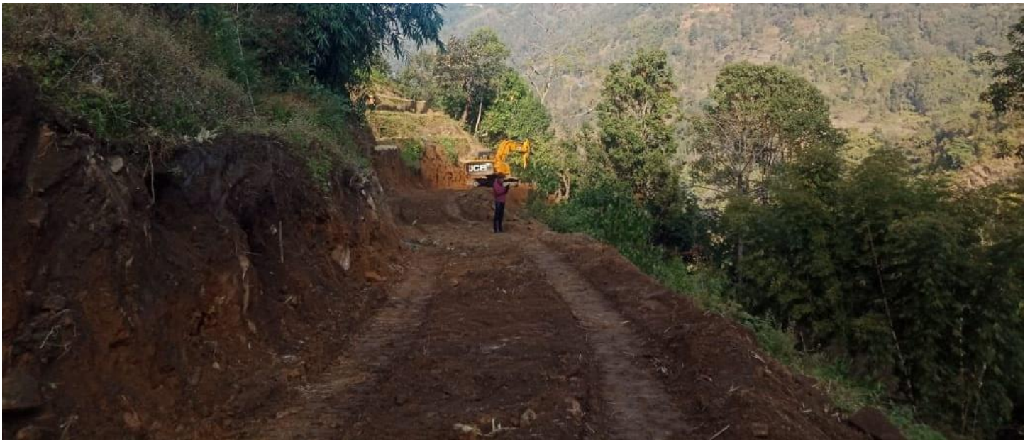
Figure 8: Construction of project road near up to surge tank
