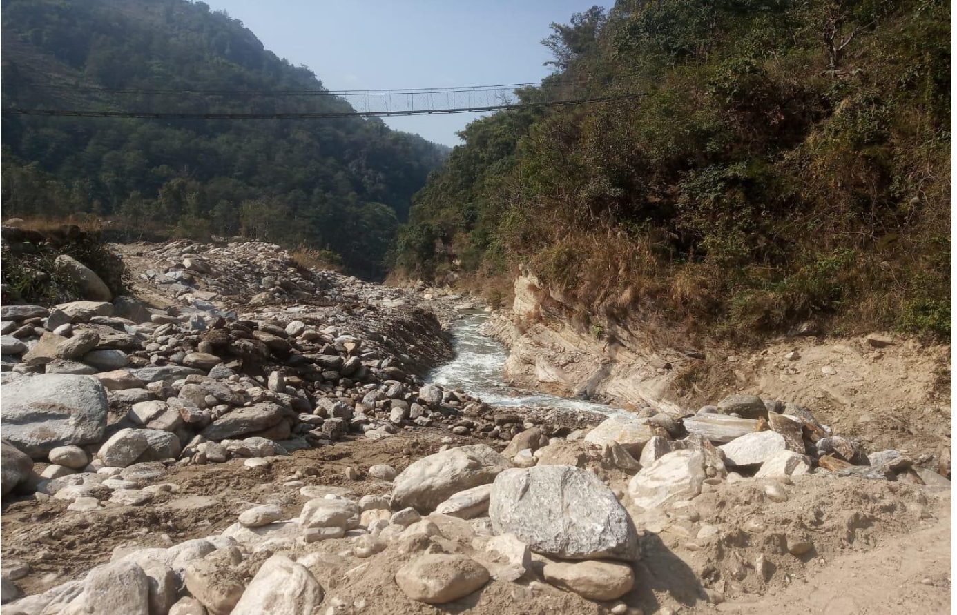
Figure 12: First Stage River Diversion
