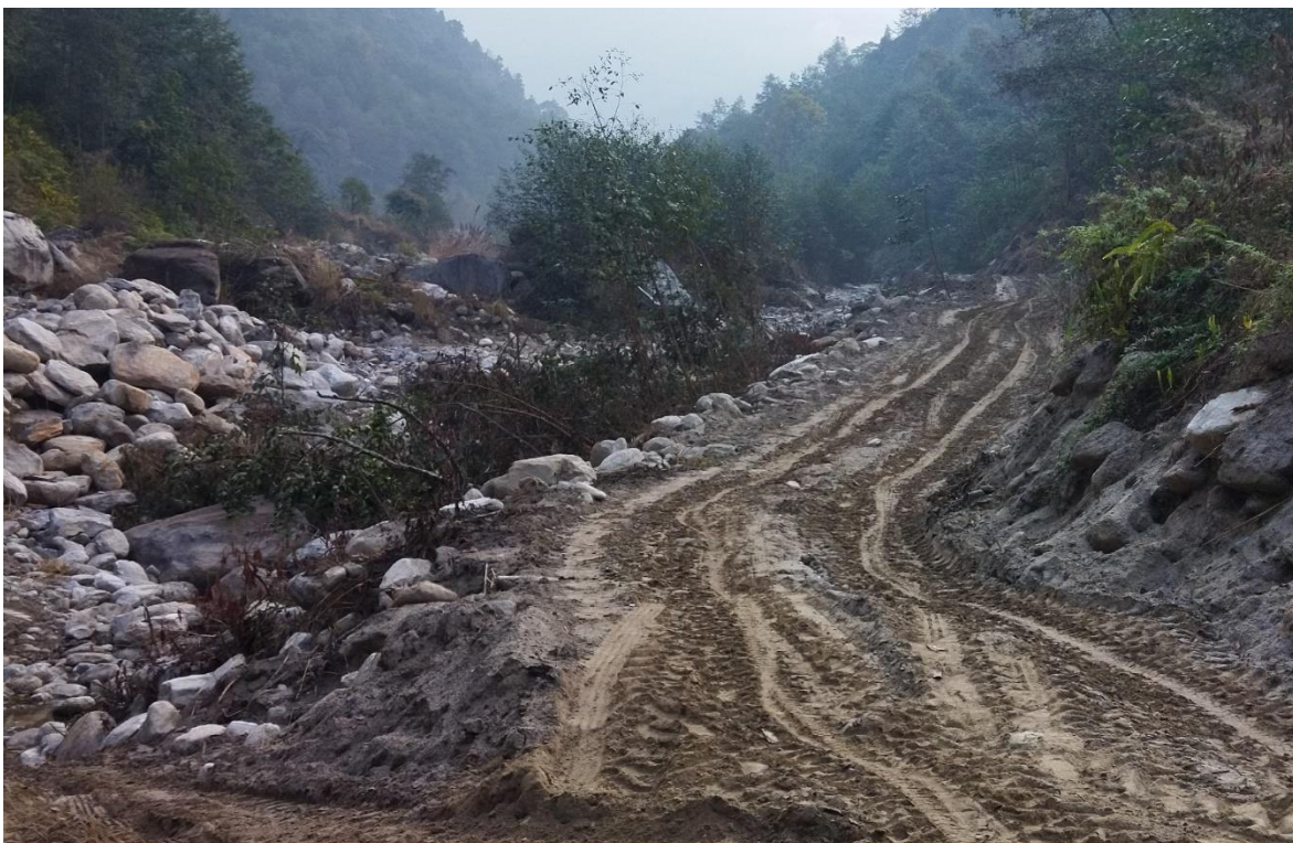
Figure 2: Access road to Headworks
