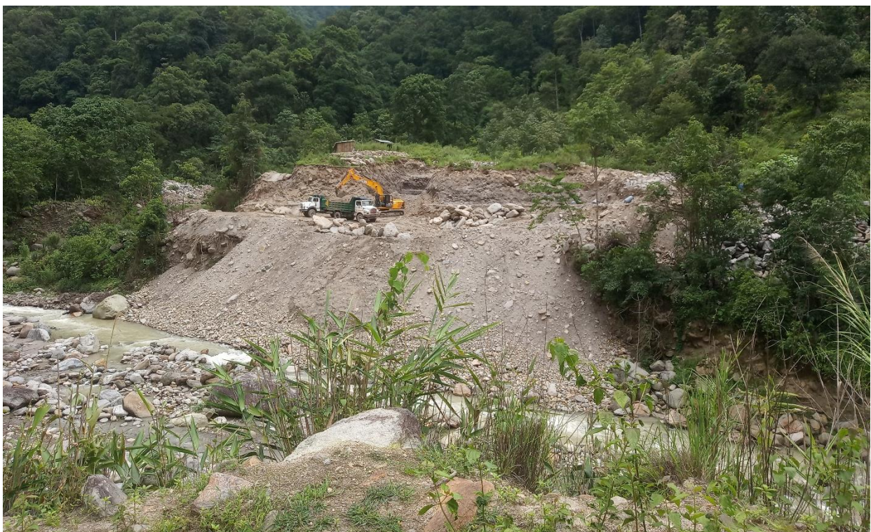
Figure 16: Excavation for Powerhouse Structures
