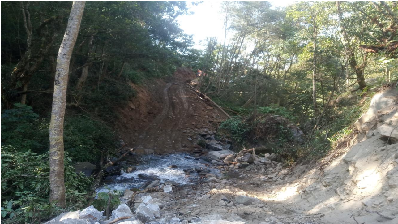
Figure 7: Construction of Project Road
