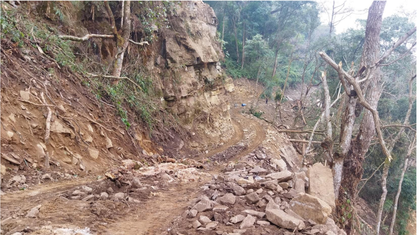
Figure 9: Construction of Project Road
