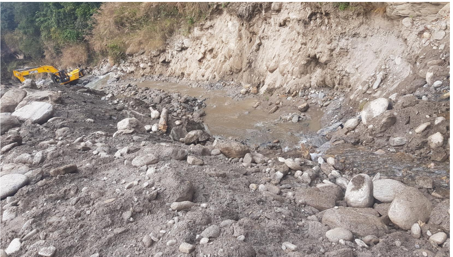
Figure 10:Excavation for First stage river diversion
